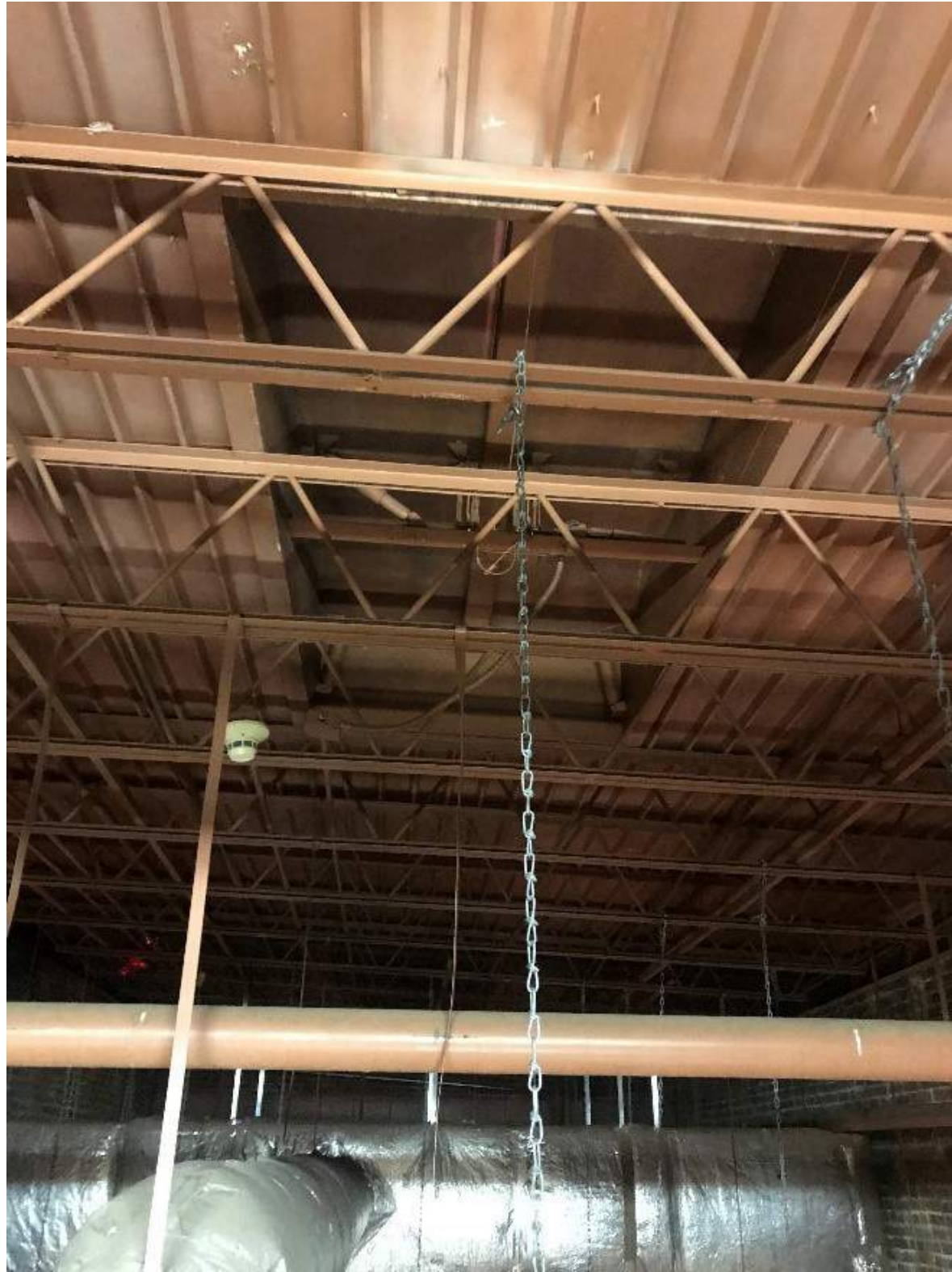
STAGE ROOF FRAMING
