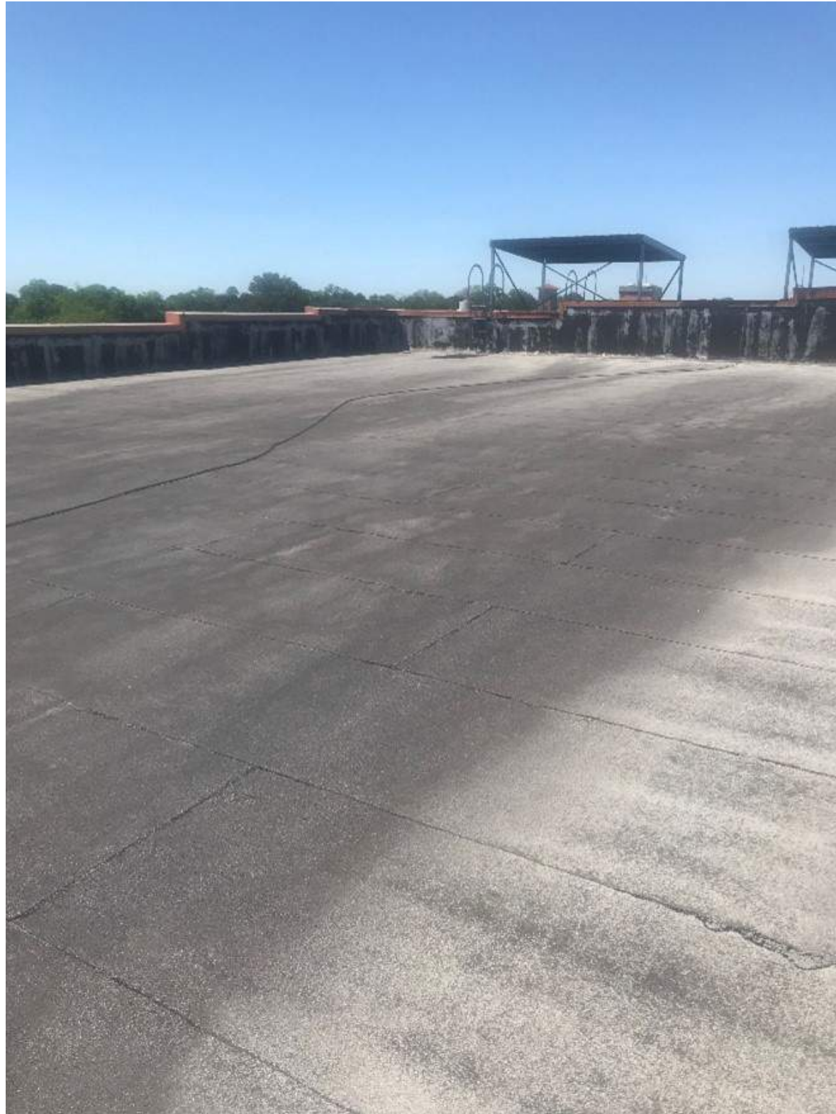
LOOKING ACROSS HOUSE ROOF
